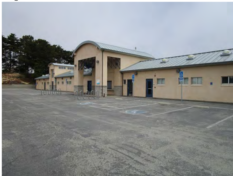
Figure 1. Main (west) elevation, looking northeast (IMG_0431)
