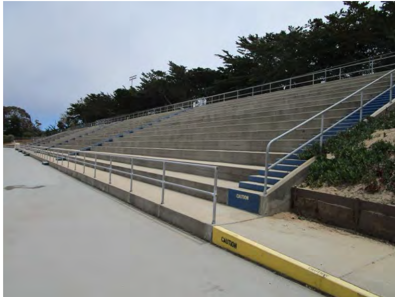
Figure 4. South bleachers, looking southeast (IMG_0434)
