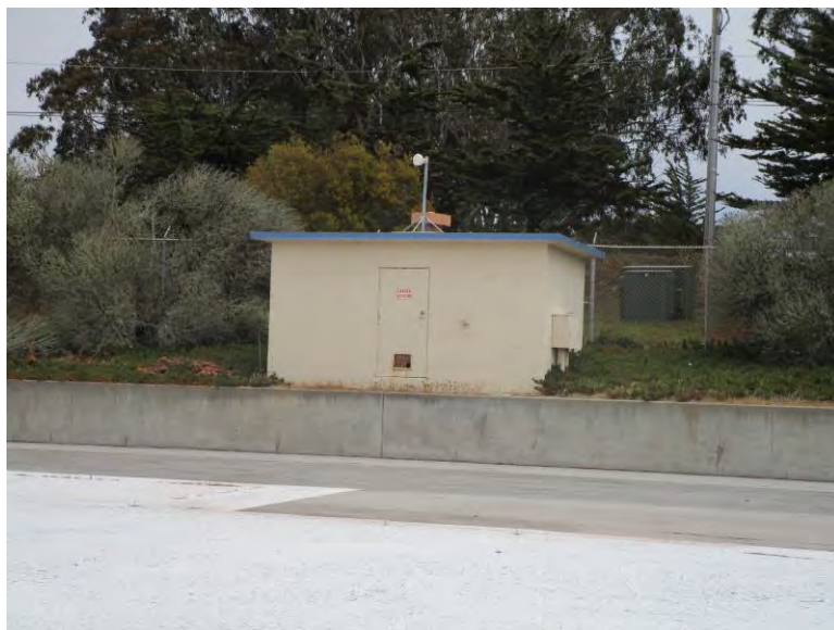
Figure 5. Electrical building, looking east (IMG_0452)
