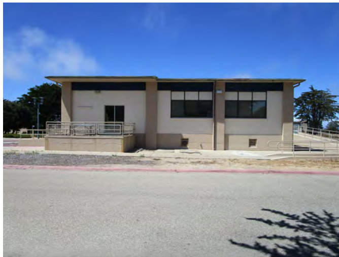
Figure 2. South elevation, looking north (IMG_0621)
