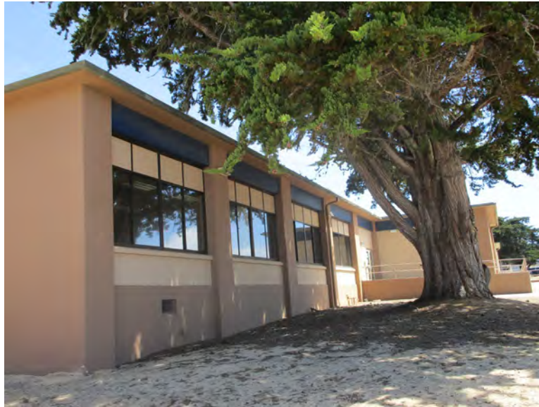
Figure 1. Main (west) elevation, looking southeast (IMG_0644)
