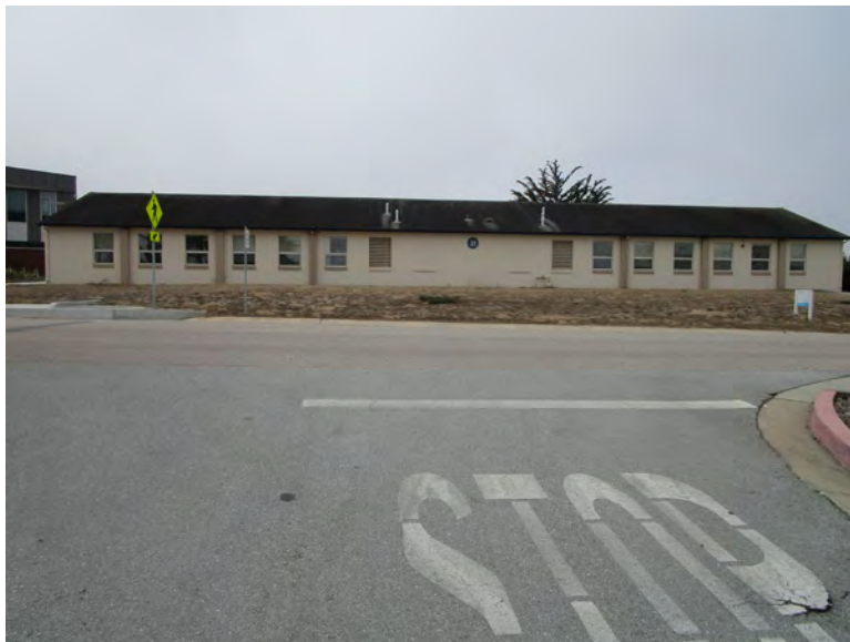
Figure 2. North elevation, looking south (IMG_0314)
