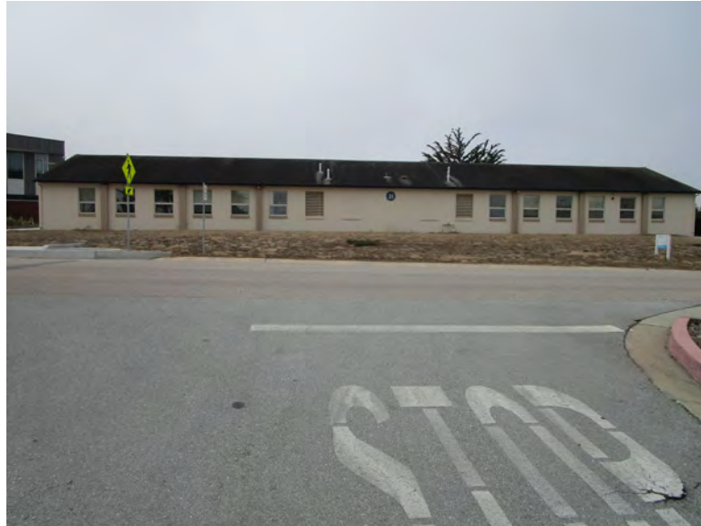
Figure 2. North elevation, looking south (IMG_0314)
