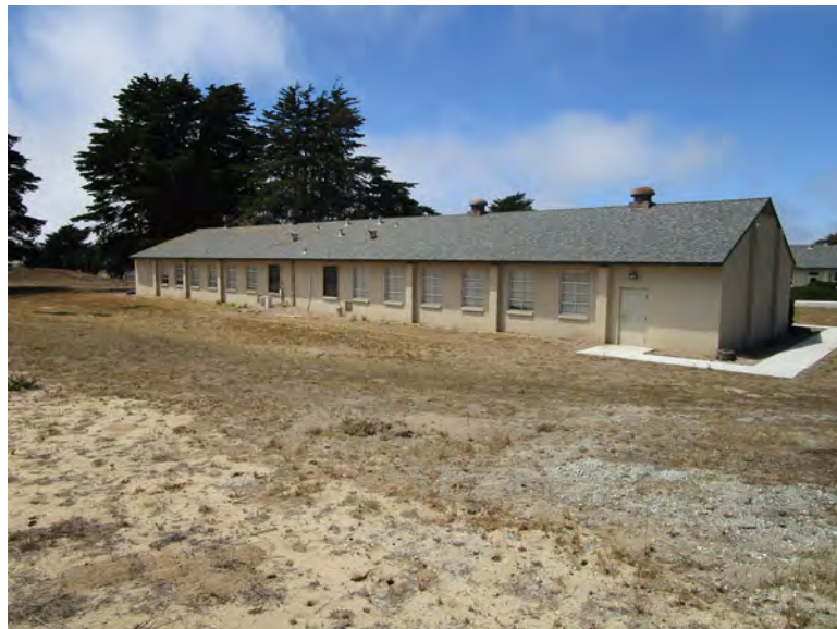
Figure 2. South elevation, looking northwest (IMG_0576)
