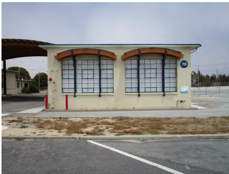
Figure 1. Main (south) elevation, looking north (IMG_0335)
