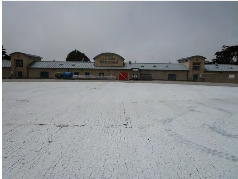
Figure 2. East elevation, looking west (IMG_0477)
