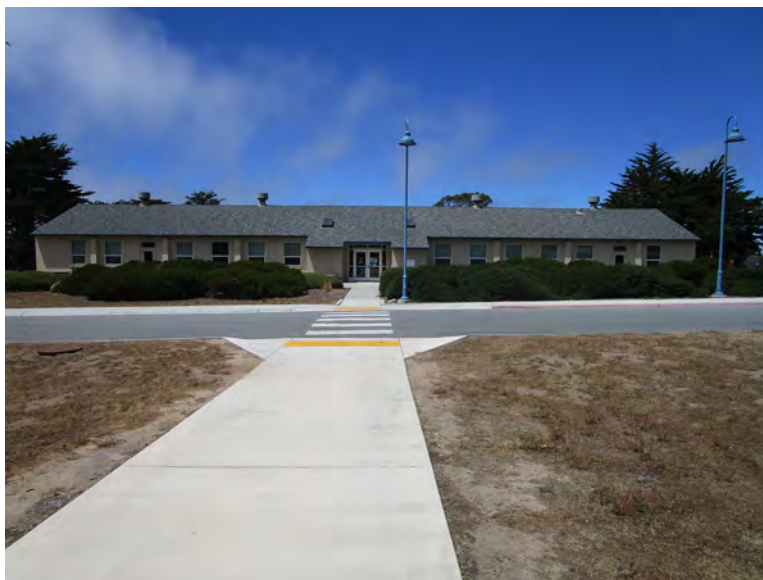
Figure 1. Main (south) elevation, looking north (IMG_0581)
