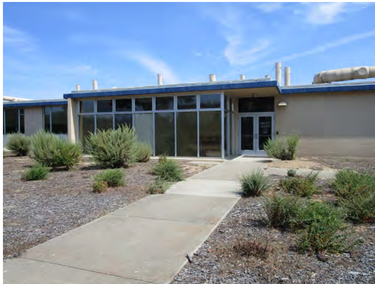
Figure 1. Main (south) elevation and entrance, looking northwest (IMG_0715)
