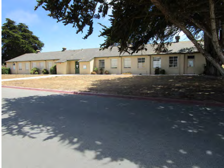
Figure 1. Main (north) elevation, looking southeast (IMG_0566)
