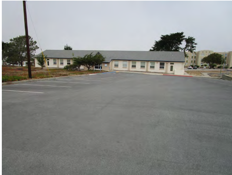
Figure 1. Main (south) elevation, looking north (IMG_0292)
