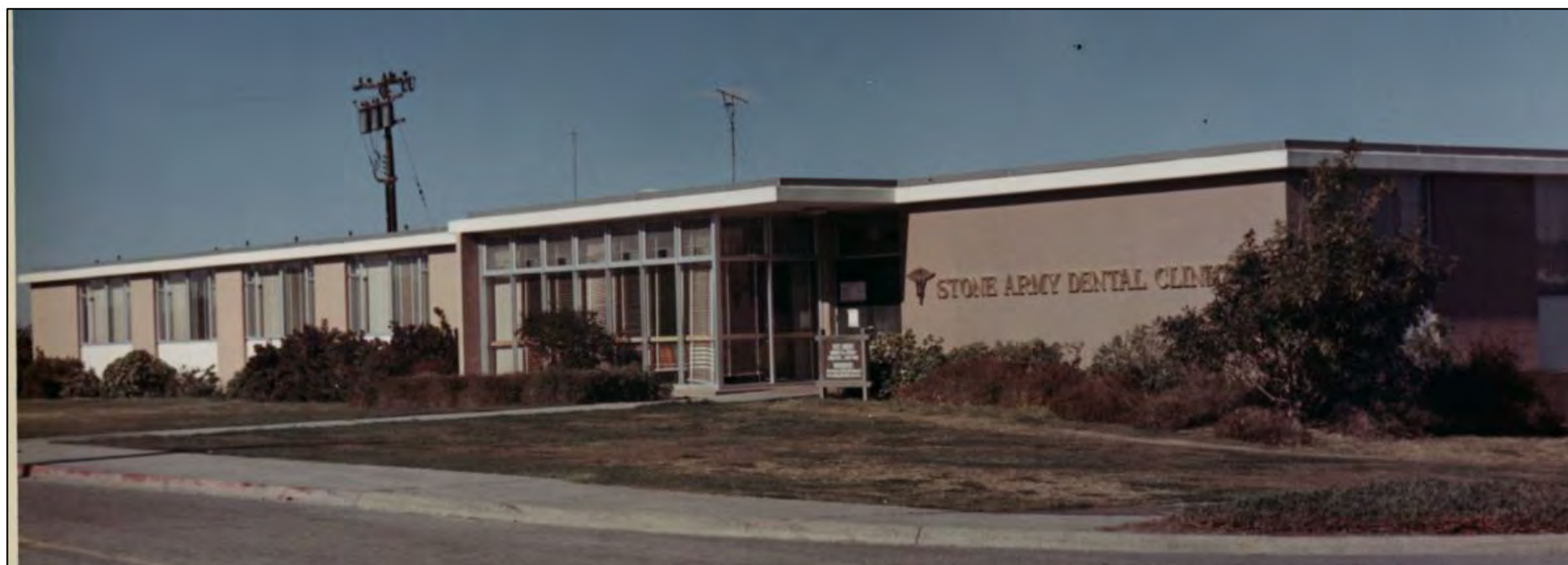
Figure 11. Photograph (c. 1990) of the Science Research Lab Annex (Building 13) after its conversion to the Stone Army Dental Clinic (DLIFLC 2021).
