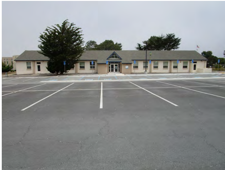
Figure 1. Main (south) elevation, looking north (IMG_0302)
