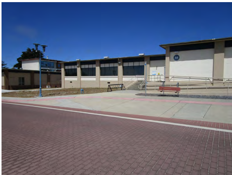
Figure 2. Main (west) elevation, looking northeast (IMG_0654)
