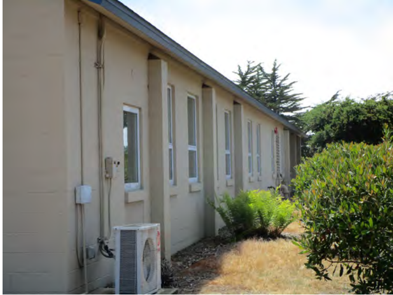
Figure 2. north elevation, looking southwest (IMG_0598)
