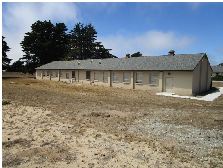
Figure 2. South elevation, looking northwest (IMG_0576)
