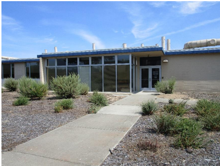
Figure 22. Building 13, the Science Research Lab Annex, View facing northwest at the south elevation (IMG_0715).
