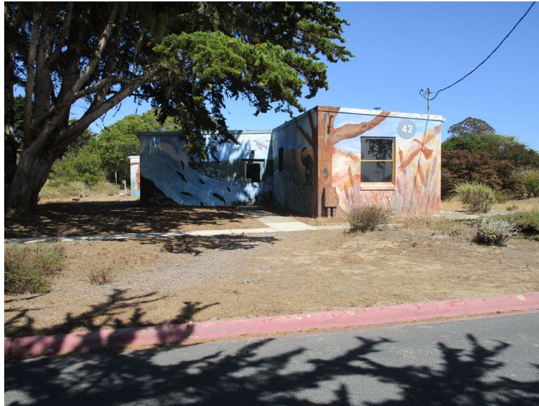
Figure 2. West elevation, looking east (IMG_0675).
