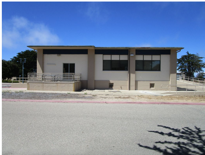
Figure 2. South elevation, looking north (IMG_0621)
