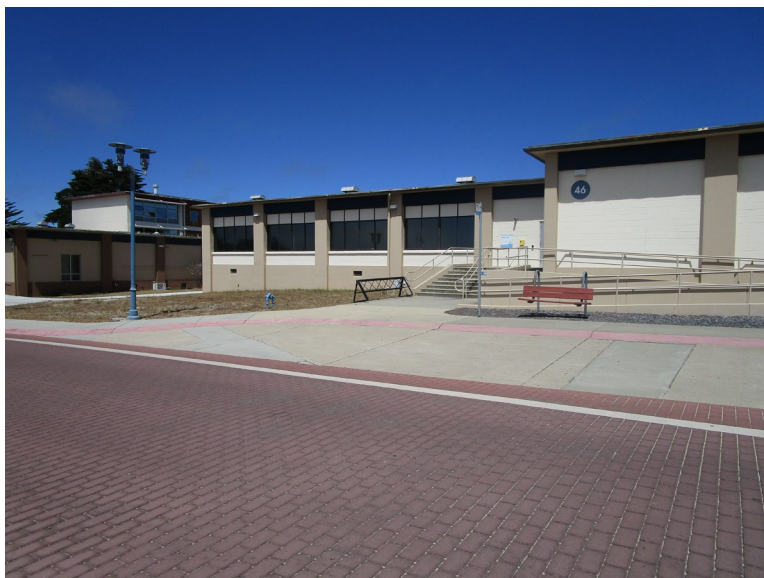
Figure 2. Main (west) elevation, looking northeast (IMG_0654)
