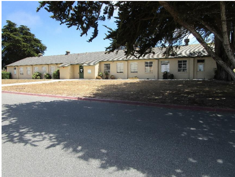
Figure 21. Building 58, Green Hall, View facing southeast at the north elevation (IMG_0566).
