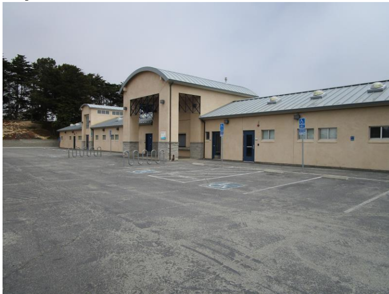
Figure 1. Main (west) elevation, looking northeast (IMG_0431)
