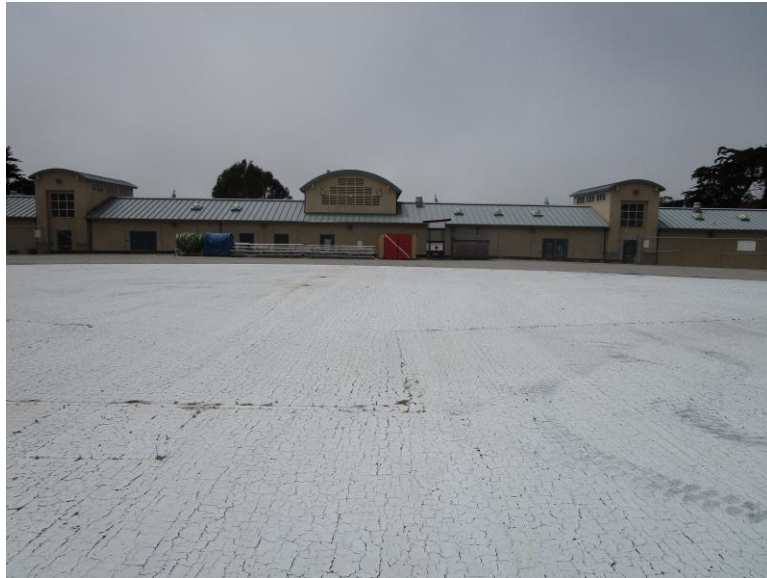
Figure 2. East elevation, looking west (IMG_0477)
