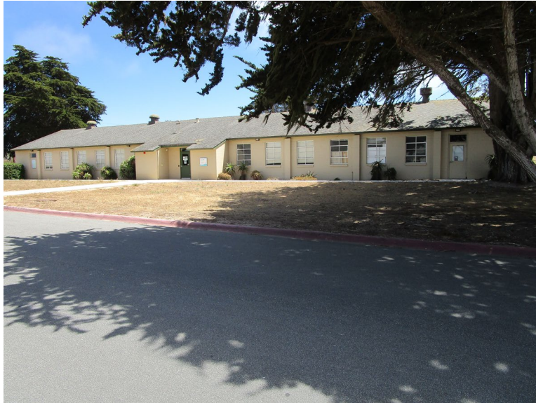
Figure 1. Main (north) elevation, looking southeast (IMG_0566)
