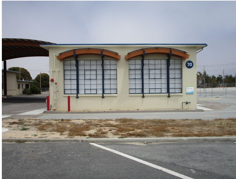
Figure 1. Main (south) elevation, looking north (IMG_0335)
