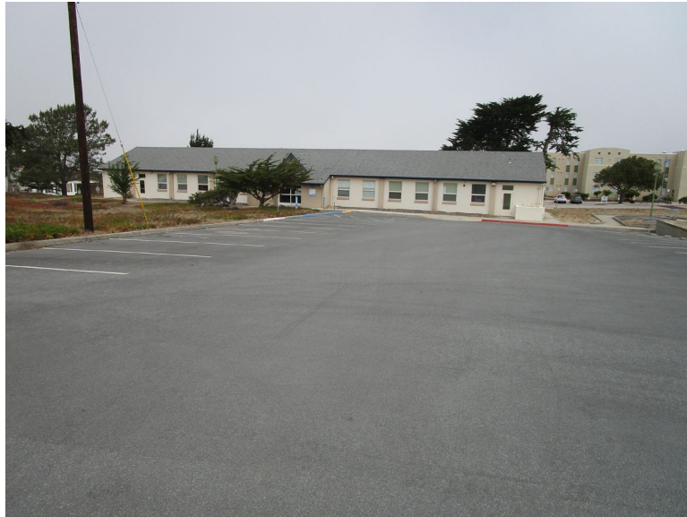
Figure 1. Main (south) elevation, looking north (IMG_0292)
