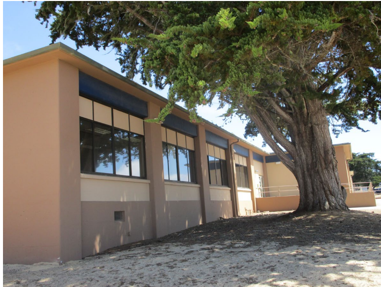
Figure 1. Main (west) elevation, looking southeast (IMG_0644)
