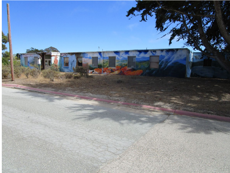
Figure 1. Main (north) elevation and entrance, looking southeast (IMG_0681)
