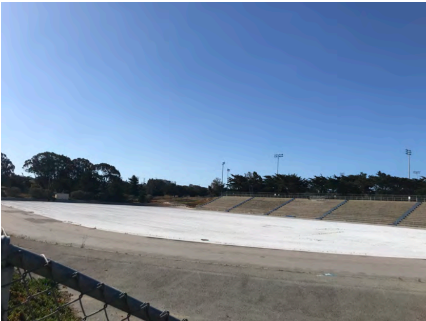
Interior project site looking southeast.
