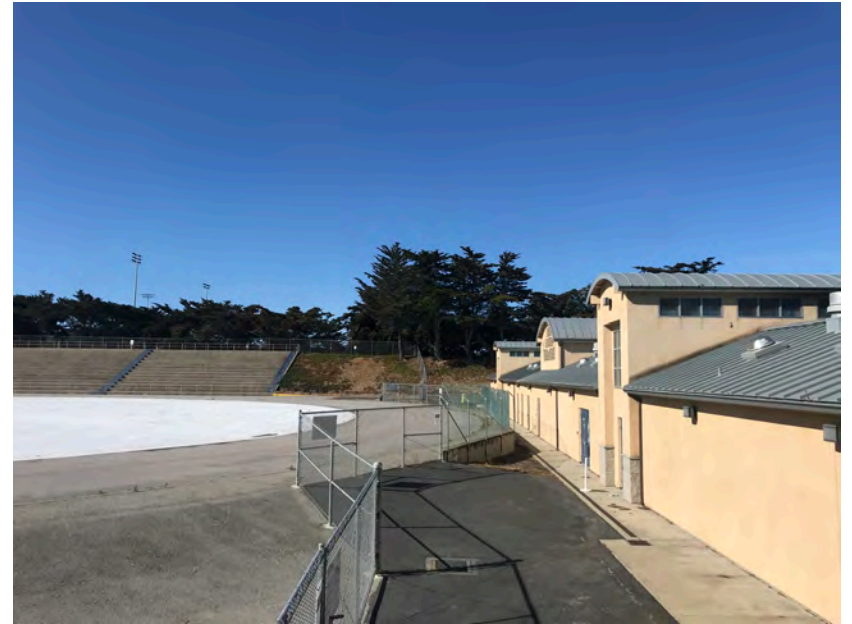
Interior project site looking south.
